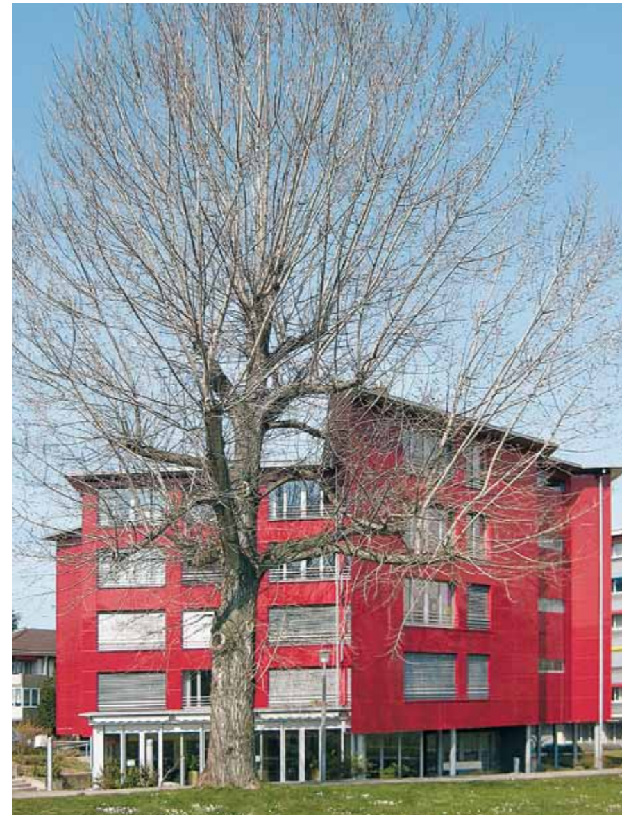
Because of its lightweight construction, Cocoon is perfect for adding storeys to existing buildings.
